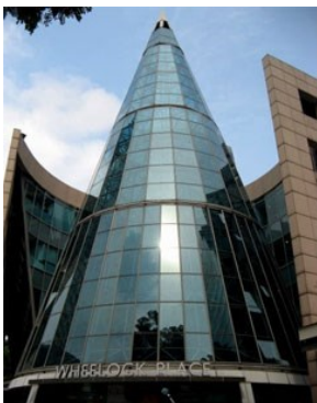
Wheelock Place Building Pitch Angles is below 90 Degree
