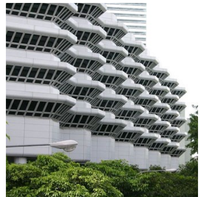
Concourse Building Pitch Angles is above 90 Degree
