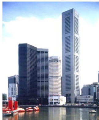
Most of building Pitch Angles are 90 Degree
