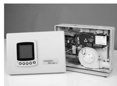
ပုံ ၈-၄၆ Air Sampling Smoke Detector with Cover Removed
