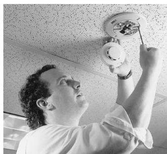
ပုံ ၈-၂၆ Technician removing wire from device to check electrical supervision
